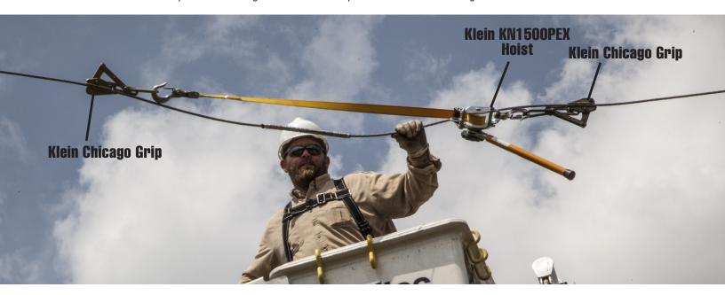
3. When finished with the splice, break the tension using the hoist handle, then use either the handle or drum knob to continue releasing the tension.
